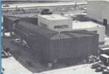
M.A.C. Low Speed Wind Tunnel Under Construction
