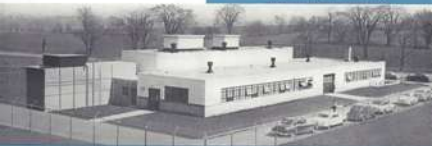
New $1,000,000 Refrigeration Laboratory at Lambert Field
